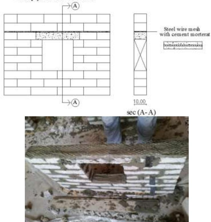
**Figure 5.** Strengthening brick walls with opening using one horizontal ply of steel wire mesh embedded into bed joint mortar above lintel.
