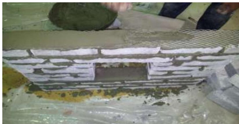
**Figure 8b . Strengthening brick walls with opening using four horizontal plies of steel wire mesh embedded into bed joint mortar (two plies above lintel and two plies at sill level)**
