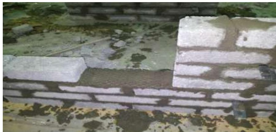
**Figure 6 . Strengthening brick walls with opening using two horizontal plies of steel wire mesh embedded into bed joint mortar above lintel and sill level.**
