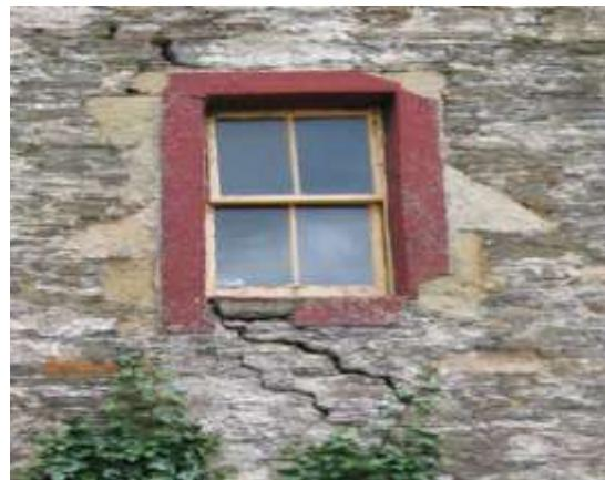
**Figure 1.** Cracks around window opening By Ingval Maxwell Published by Technical Conservation Group
