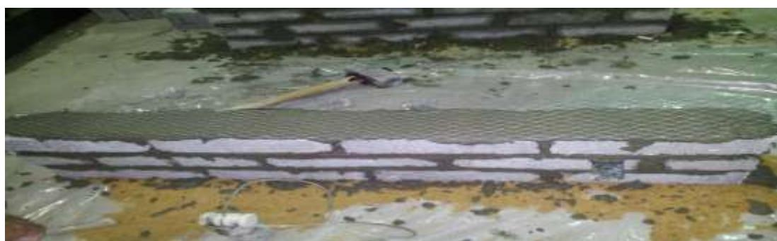
**Figure 9. Steel mesh used into bed joint mortar**
