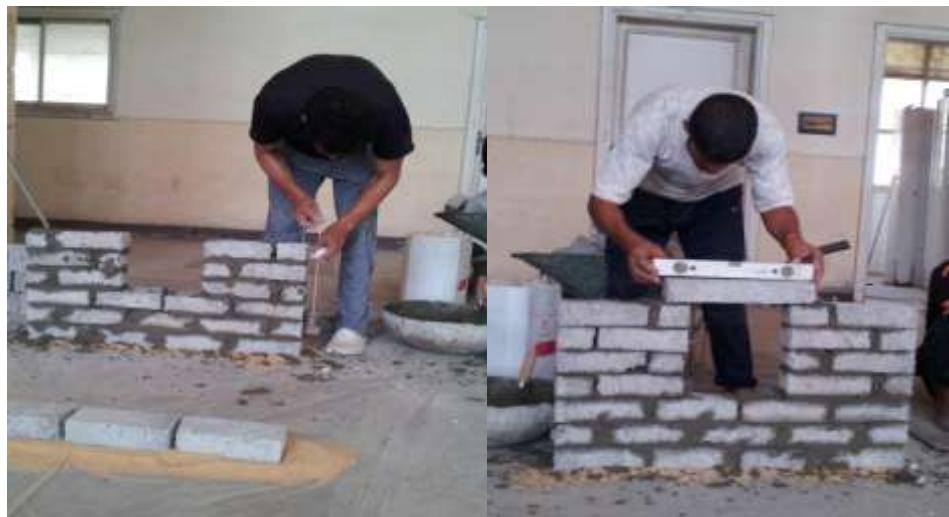
**Figure 3.** Brick wall specimen during construction
