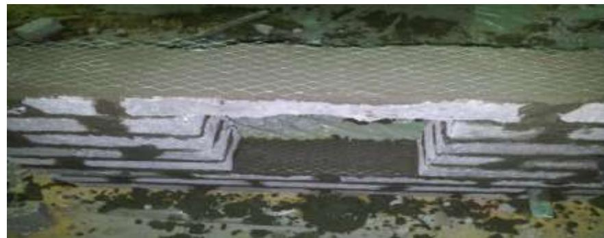
**Figure 7.** Strengthening brick walls with opening using three horizontal plies of steel wire mesh embedded into bed joint mortar (two plies above lintel and one ply at sill level)
