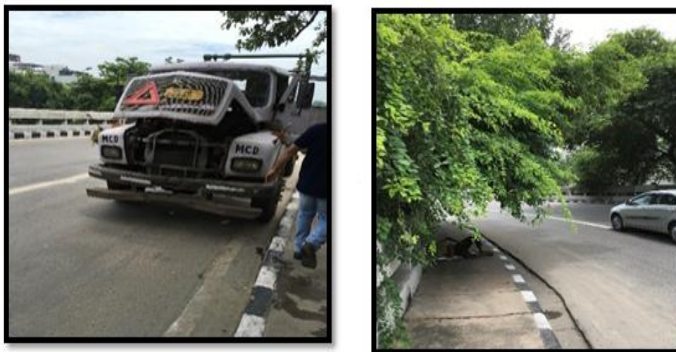
Figure 10 Heavy truck parked on the acceleration ramp & bushes causing the blind spots during acceleration operation and it has a sharp curve
