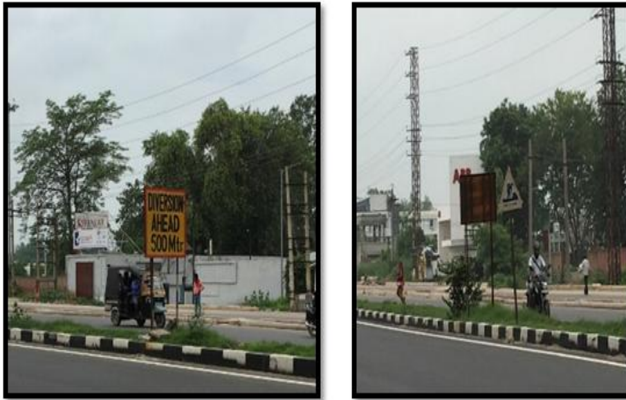
Figure 5 Sign boards without retro-refractory background & Men at Work is faded not visible clearly
