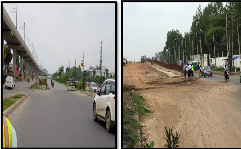
Figure 4 Open Entry to construction site
