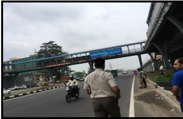
Figure 3 The column of the foot over bridge near to the carriage way
